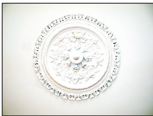
The original ceiling medallion of this home, built in 1865, is a nice architectural detail.
